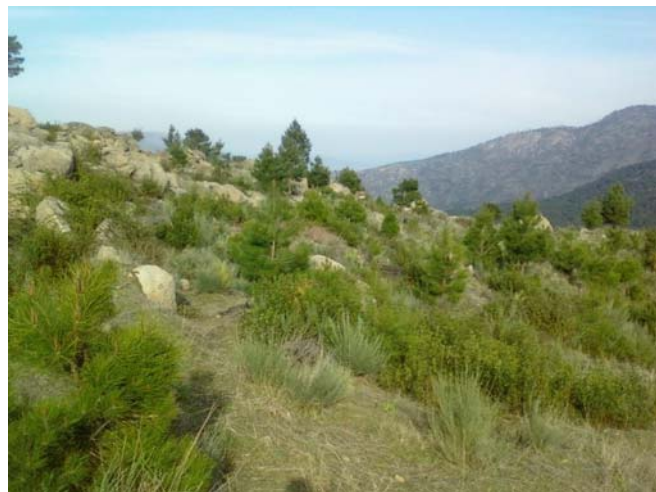
Image 6 Site 6 Valle Iruelas: Hole digging reforestation by excavator machine
